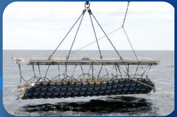
Mats are installed using our Exclusive Deployment Frame. Above: Mat supported from frame on chains.
